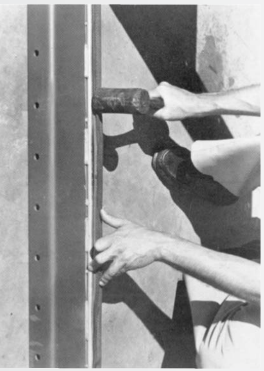
Replacing Seal
